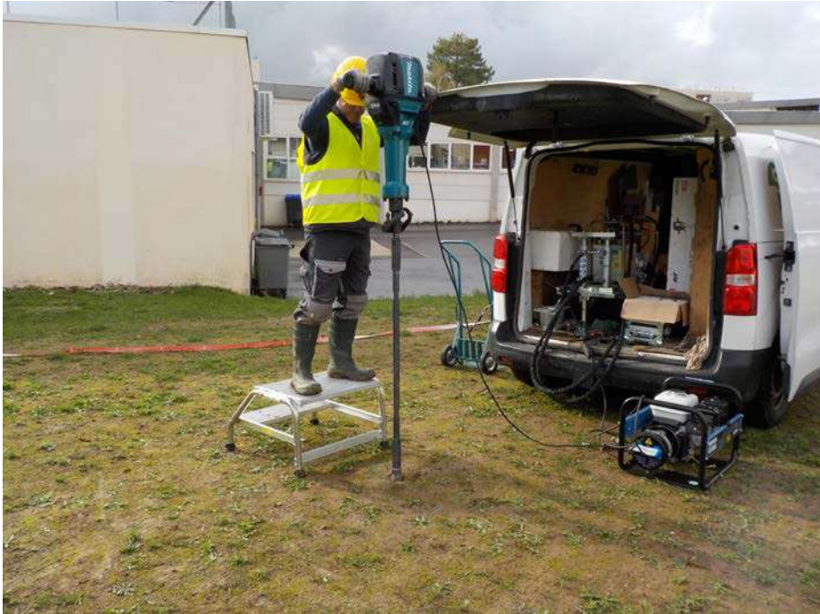
Figure 1 - Intervention au carottier portatif
